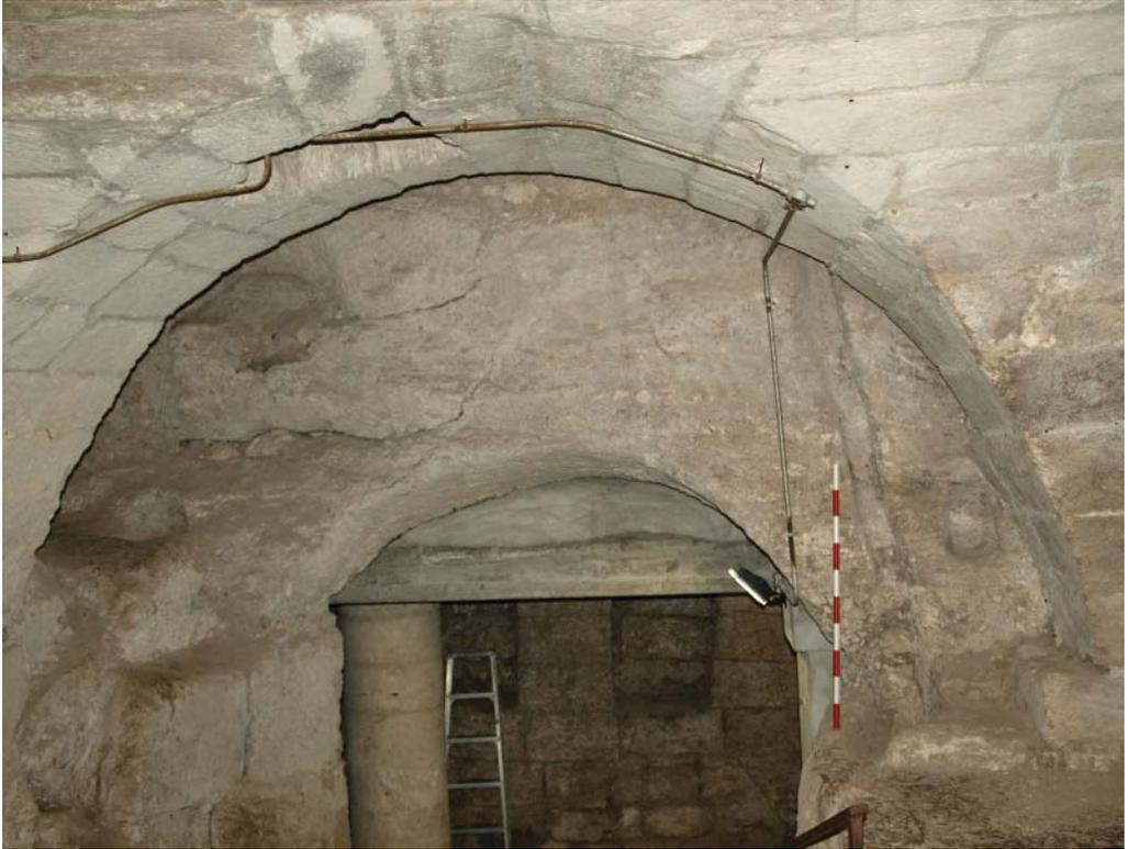
Fig. 4. The rock-cut arch opening into the Large Cave, showing by the scale a water channel cut into its face, from the east. The niched wall can be seen in the background; the cross-vault above the entranceway in the upper part of the foreground. The scale is 1m high in 10cm divisions.
