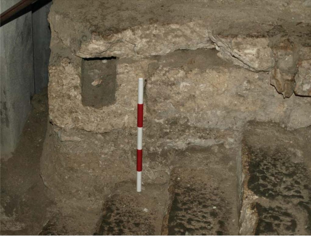
Fig. 5. The stone conduit below the later mortar floor on north-west side of the stairs into the Large Cave, from the south. The scale is in 10cm divisions.
