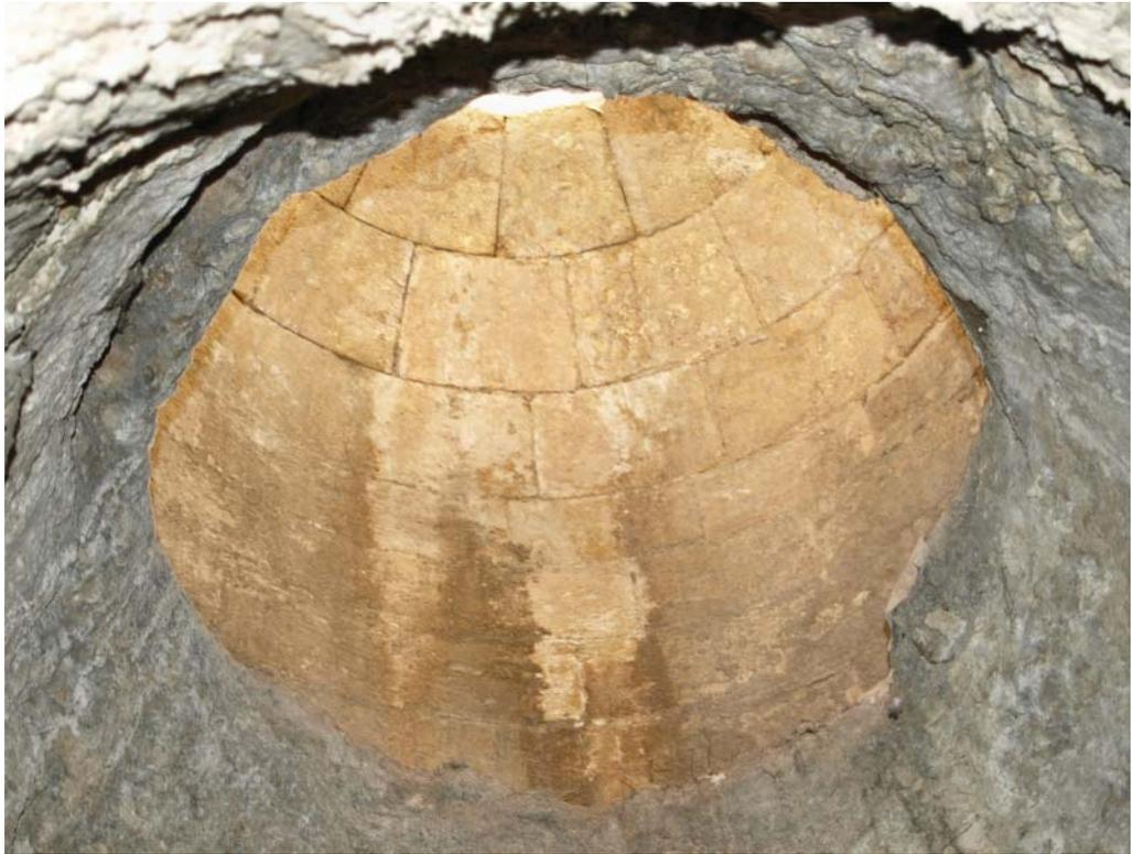
Fig. 3. The 'light well'. The earlier rock-cut aperture is encased in later Crusader-period ashlar.
