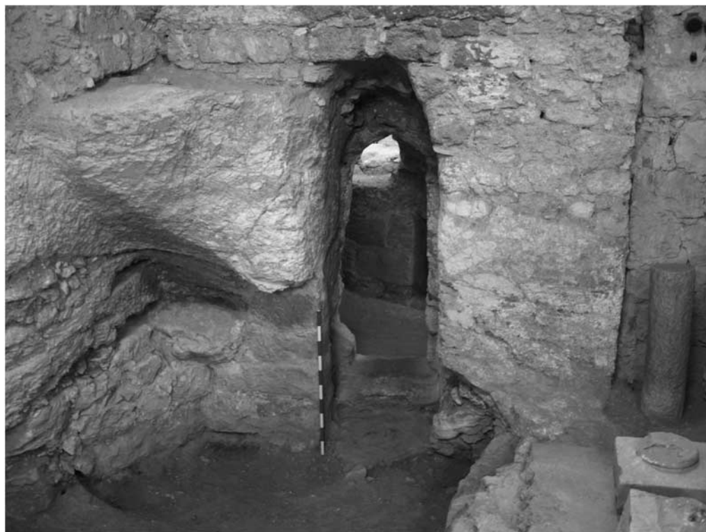
Fig 10. Structure 1 with the part of the twentieth-century concrete floors removed in 2010, from the south. The 1945 pit, seen in figure 9, is left partially filled with twentieth-century hardcore, the removal of which was unnecessary for the concrete floor to be restored. The scale is 1m high in 10cm divisions. Photograph: author
