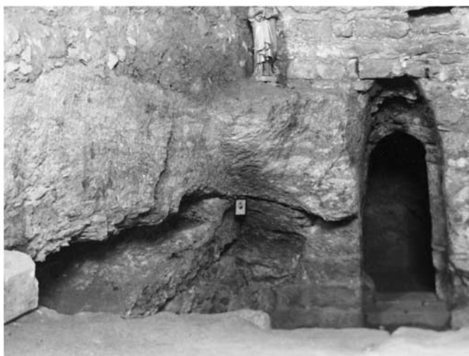
Fig 9. An anonymous photograph of 1945, showing the pit dug within the floor of Structure 1, from the south. Photograph: by permission of the Sisters of Nazareth convent
